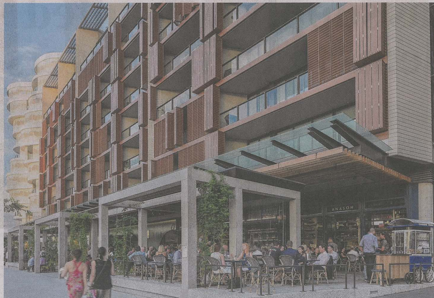
The Barangaroo South urban renewal project has been lauded for its design and sustainability features
